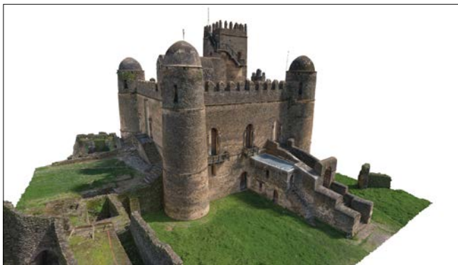
From lidar point cloud to final 3D model of Fasil's Castle, the palace of Emperor Fasilidas, in the Fasil Ghebbi fortress in Ethiopia. Once the Zamani Project team have completed the laser scanning, photography and other survey work on site, an enormous amount of post-processing is required to create the 3D models and other digital products, including plans, sections, panoramic tours and video animations.
