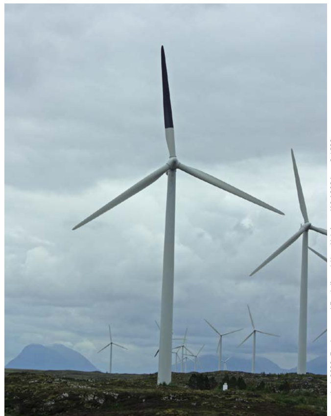
A study in Norway showed that the annual fatality rate at wind turbines with one blade painted black was reduced by more than 70% compared to neighbouring turbines.
