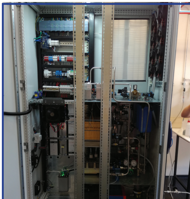
Fuel cell system installation at Poelano Secondary High School in Ventersdorp providing off-grid electricity for ICT and lighting to the school.
